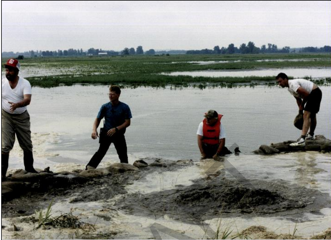
Figure 0-8. Attempts to sandbag a sand boil at the Kaskaskia Island Levee. This containment attempt was not successful, and the levee breached minutes later (Photo courtesy of USACE St. Louis District).
