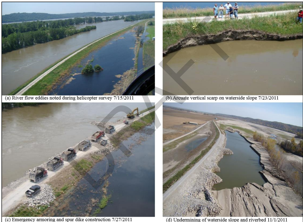
Figure 9-9-1. Missouri River Levee System (MRLS) 488-L during and after the 2011 Missouri River Flood (Photos by USACE Kansas City District).
